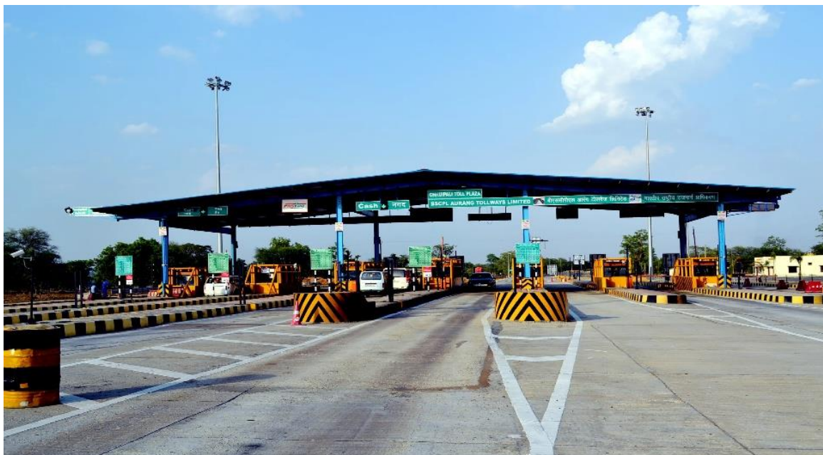
Chhuipali toll Plaza, Chhattisgarh
